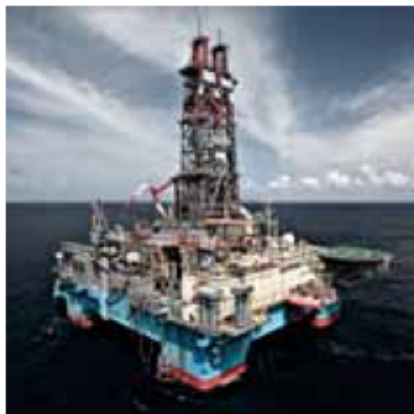
DPS2/M, column stabilised dynamically positioned semi-submersible
